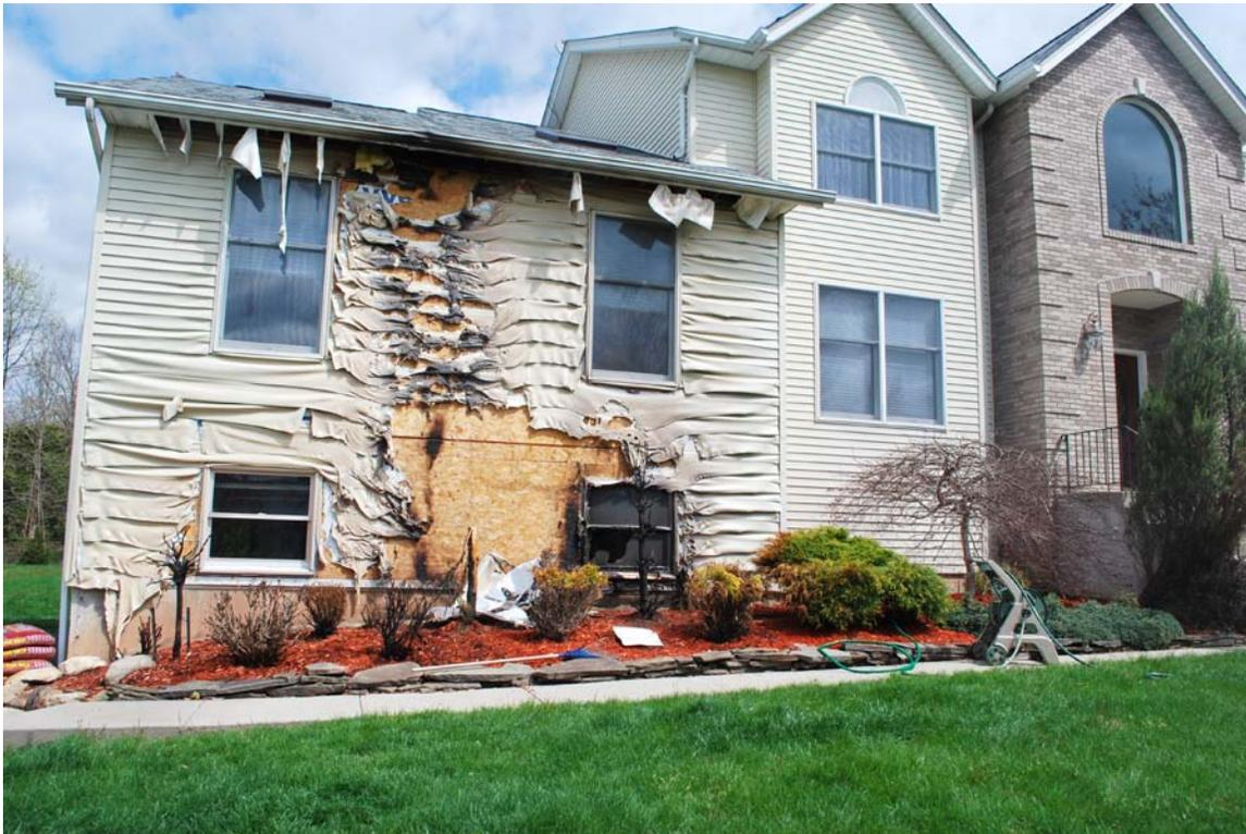
We conducted some experiments with the actual offending mulch. Our results indicated that once fire is introduced to the dry mulch it smolders for about one minute and then there is rapid ignition along the top of the mulch. A strong breeze is a plus in the spread of the flames.
